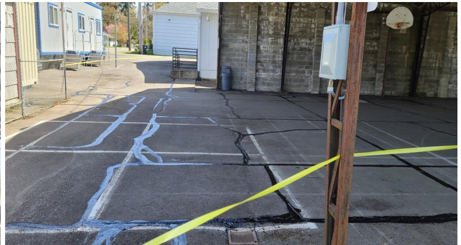
Cracks Repaired
